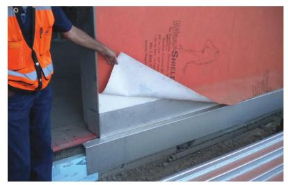
Figure 3: An example of wall to roof transition with material compatibility issues.
