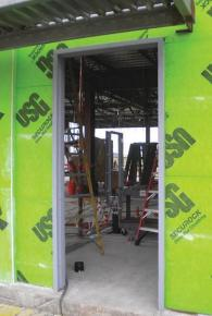
Figure 2: Here is an example of an untreated rough opening. A preconstruction meeting could have prevented this issue.
