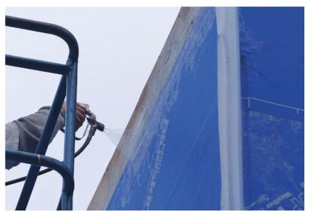
Figure 1: An example of primer being applied to the face of a polyolefin membrane.
