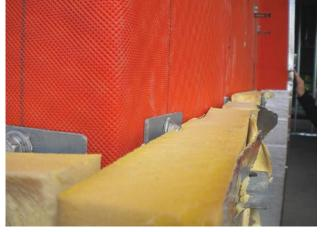
Figure 5: An example of a wall installation with an improperly designed rain screen. Note the rigid insulation installed directly over the face of the WRB/AB preventing proper drainage.
