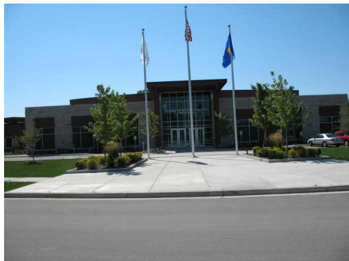
VaproShield WallShield Black was installed on the Mt. Pleasant Village Center.
