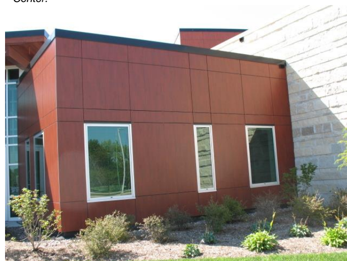
WallShield was installed behind Trespa phenolic rain screen system.
