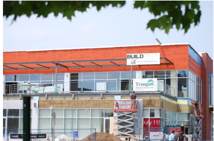
Over 5,000 sq. ft. of WrapShield SA Self-Adhered used on multi-use building.
